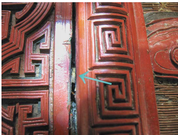
Fig. 17: Bamboo dowel between the inset panel and frame.
