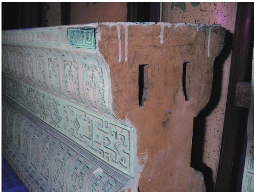
Fig. 40: Secondary coating in UV light, with drips.
